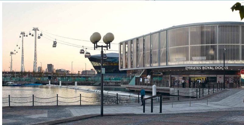
The dedicated carrier for sheave assembly replacement was used for the first time in March 2016 in London and then in Singapore in September.
